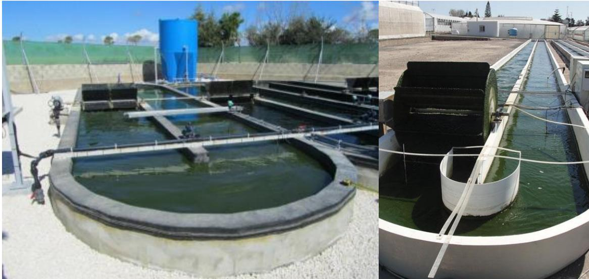
**Figure 5.3. A HRAP produced by Aqualia and used for wastewater treatment.**
