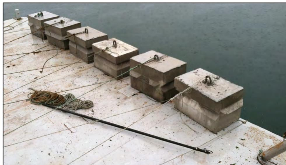
**Figure 1.5 Concrete block moorings**
